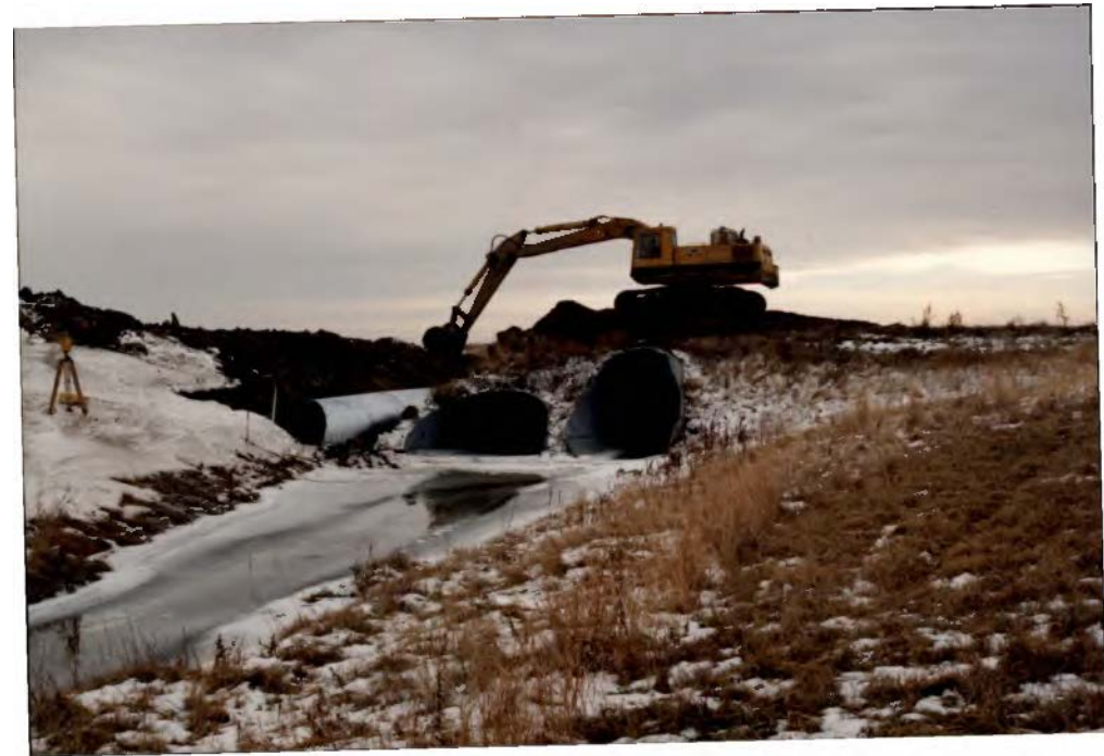
Added 8-foot circular pipe in 1995
