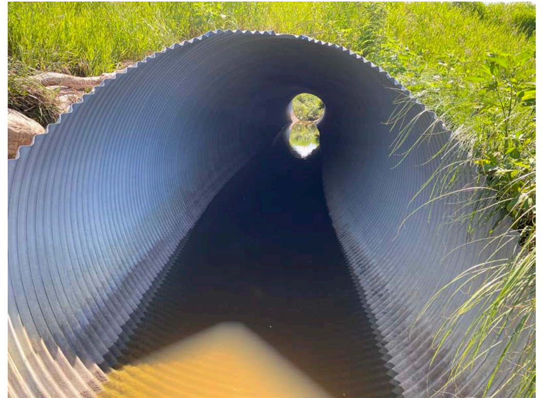
North east pipe: 8-foot circular pipe is in good shape.
