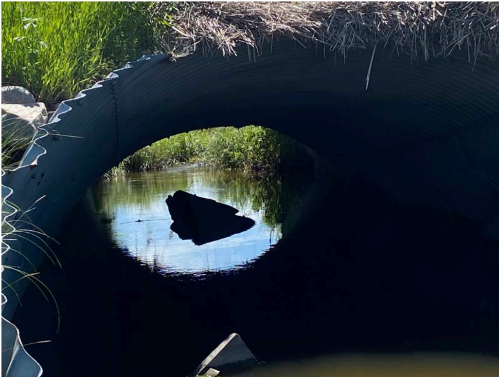
Center pipe: 9'5" x 15'6" SPPA is buckling on bottom and caving in on top.
