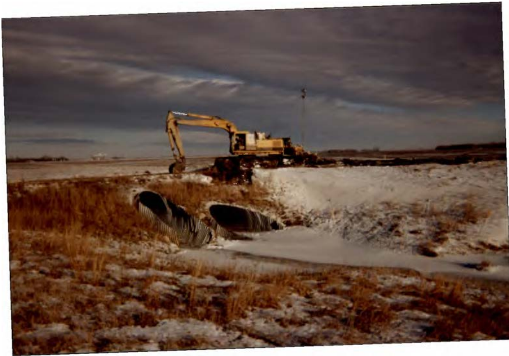
Before adding additional pipe in 1994
